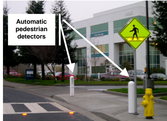
Example in-pavement crosswalk lights and automatic pedestrian detectors
