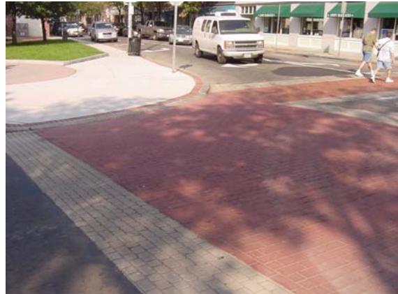
New curb cuts and new faux brick crosswalks provide safe pedestrian access while complimenting the historic area.
