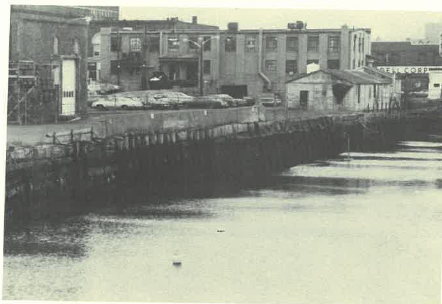
Bulkhead on south side of channel at Massachusetts Electric Company. Note concrete "safety" wall installed opposite garage entrance door and steel sheet fender piles in channel formerly used to tie up vessels away from granite wall.
