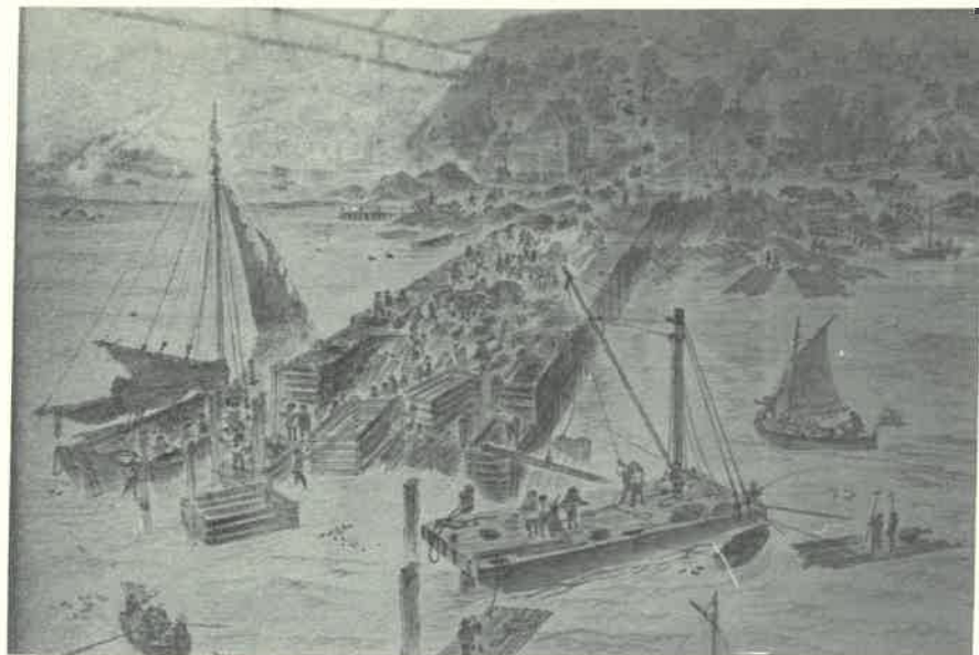
Pier is built as wooden cribs are floated into place between piles and filled with stone brought in wagons.
