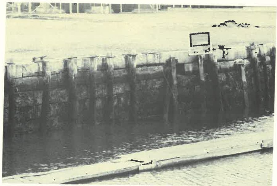
Typical granite block bulkhead. Segment shown is on south side at Mass. Electric abandoned coal storage site.
