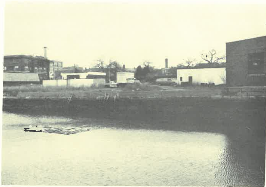
North bulkhead at rear of Derby Street Texaco Station. Note cement concrete header wall and "trueness" of joints in granite block wall despite heavy building surcharge.
