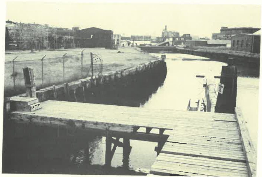
The South River Channel from the Congress Street Bridge. Wooden Wharf in foreground is used by lobstermen. Note steel sheet pile bulkhead (c. 1941) and twin conduits at far (west) end of channel.
