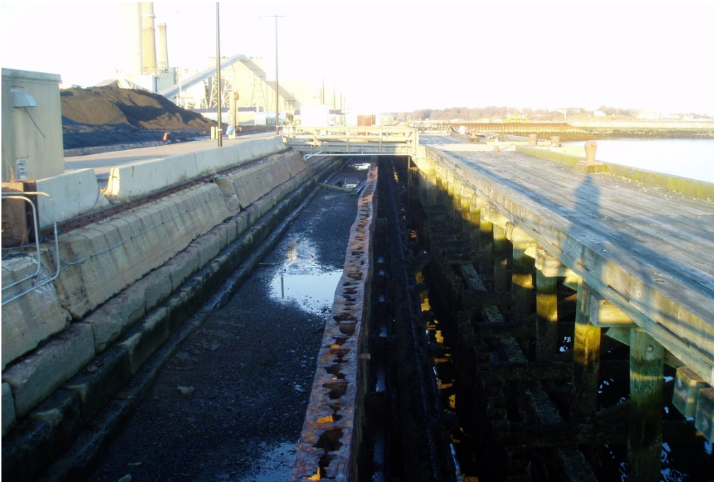
Photo 5- Looking northeast along the gap to be spanned with precast concrete or timber decking using existing supports
