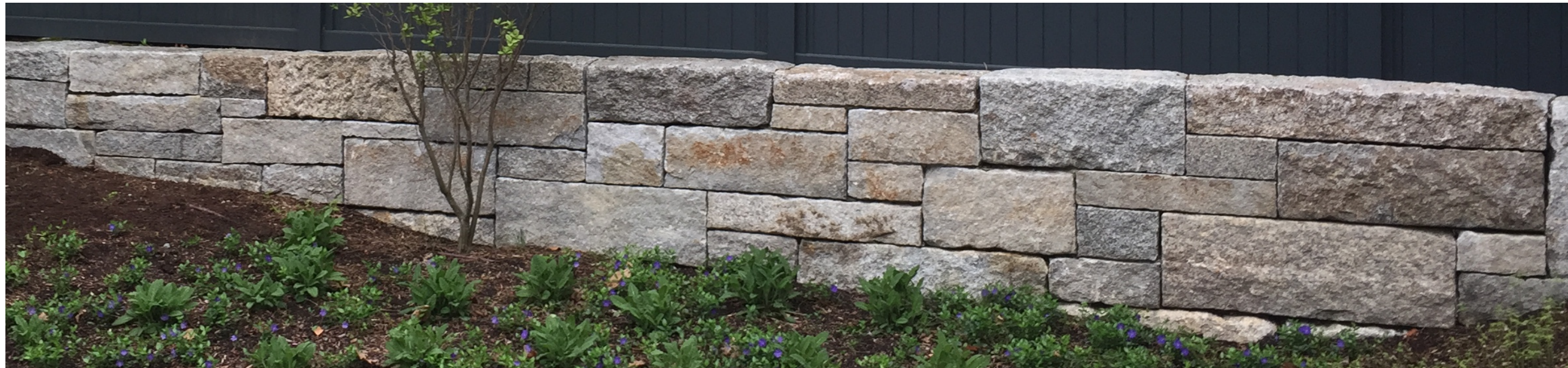
5 GRANITE RETAINING WALL (W-GR) - CHARACTER PHOTO NTS
