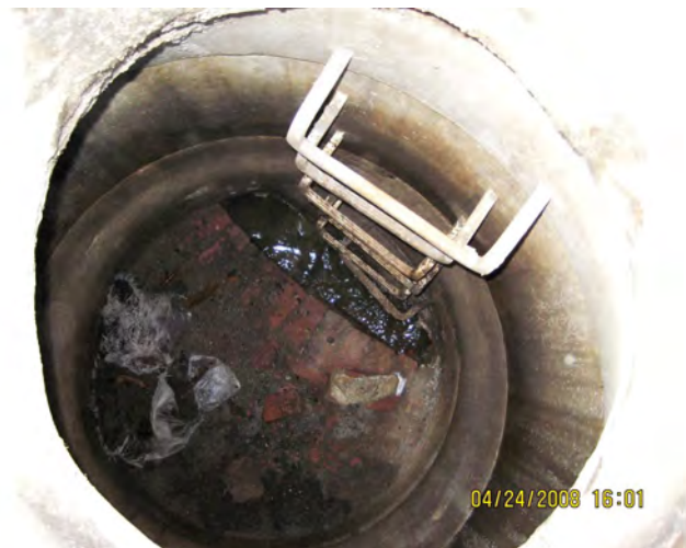
Location 35—Rebuild Invert & Bench
