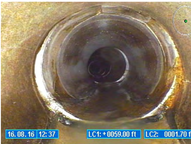
Location 43—(4-foot Repair) CIPP Spot Liner or Furnish and Install New Pipe Section
