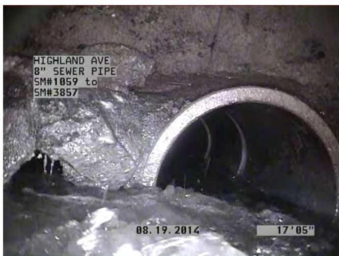
Location 57—Rebuild Invert & Bench
