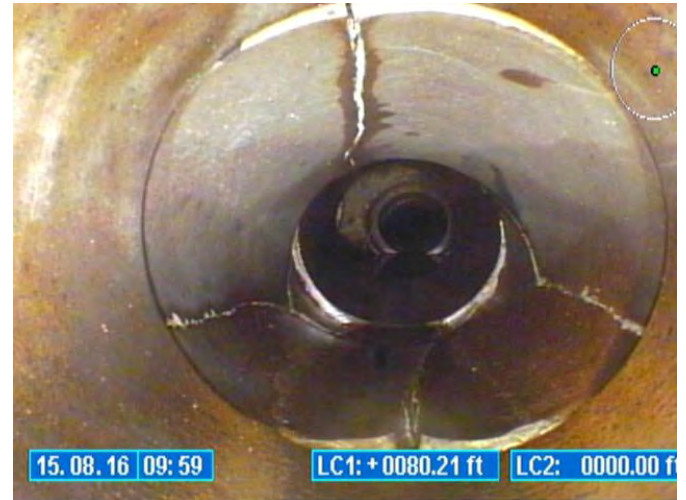
Location 42—(12-foot Drain Repair) CIPP Spot Liner or Furnish and Install New Pipe Section
