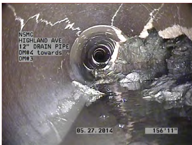
Location 59—CIPP Liner (Drain) 194-feet
