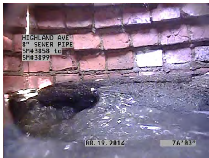
Location 47—Rebuild Invert & Bench
