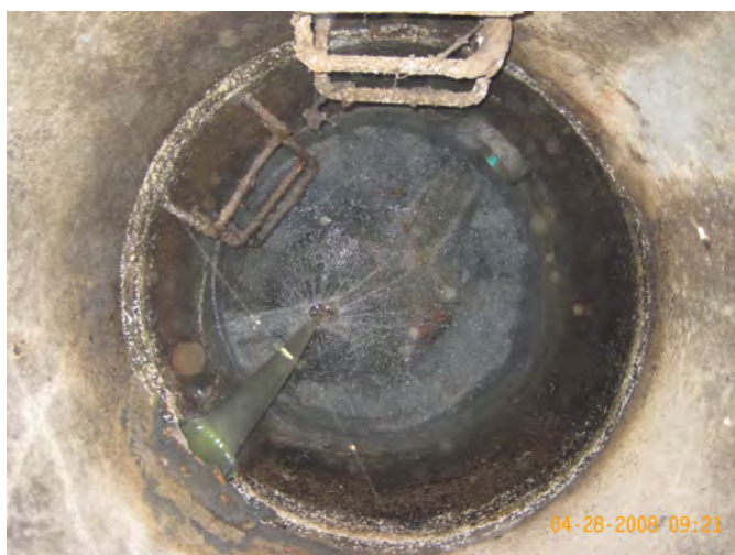
Location 33—Install 8-inch Inside Drop, Rebuild Invert & Bench
