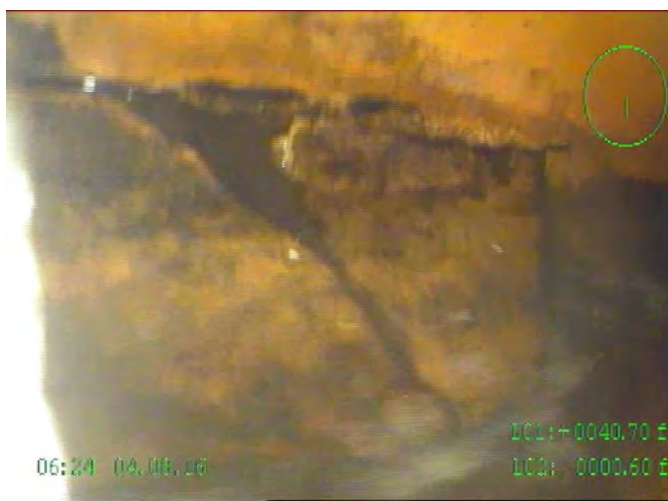
Location 31—(4-foot Repair) CIPP Spot Liner or Furnish and Install New Pipe Section
