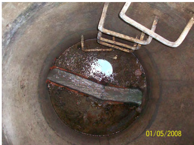
Location 37—Rebuild Invert & Bench
