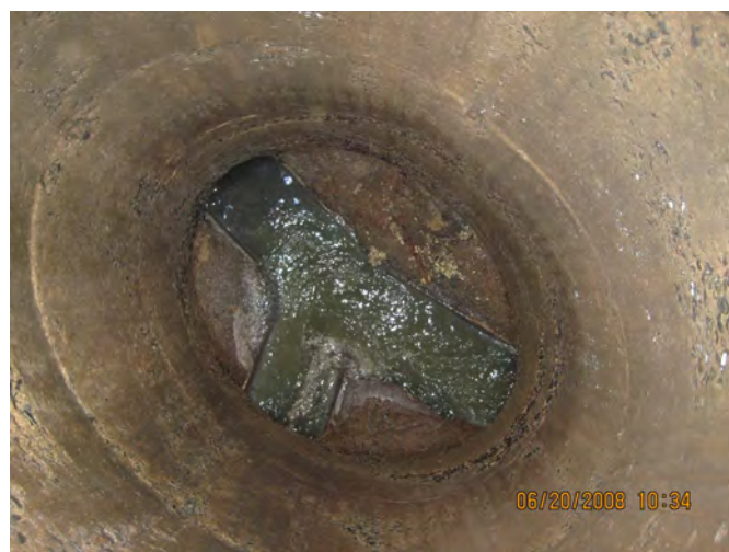
Location 58—Rebuild Invert & Bench
