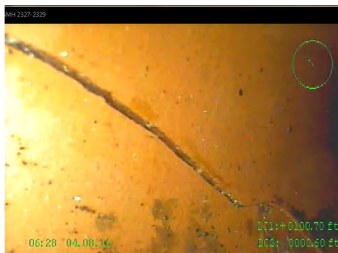
Location 32—(4-foot Repair) CIPP Spot Liner or Furnish and Install New Pipe Section
