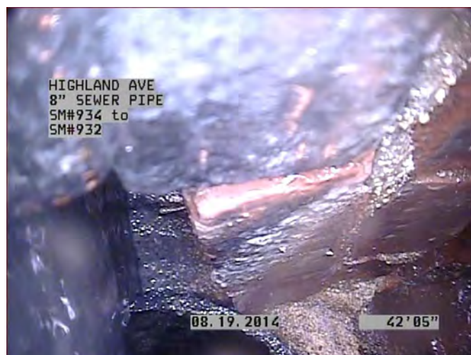
Location 46—Rebuild Invert & Bench
