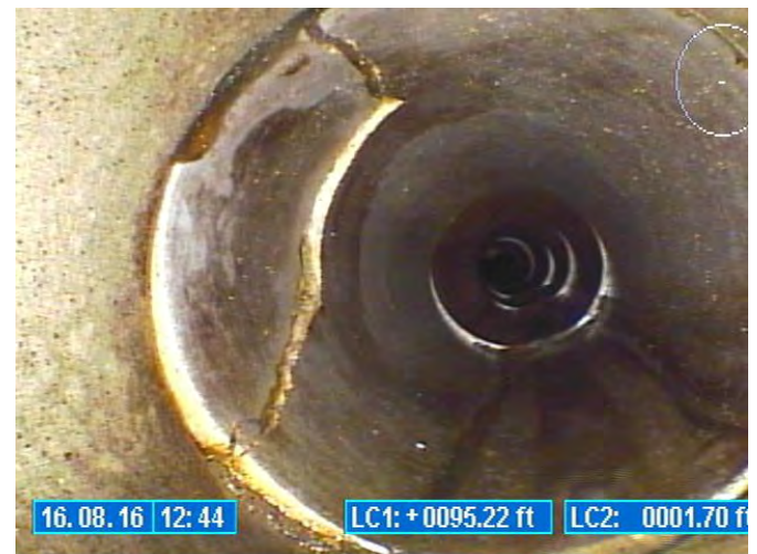
Location 44—(4-foot Repair) CIPP Spot Liner or Furnish and Install New Pipe Section
