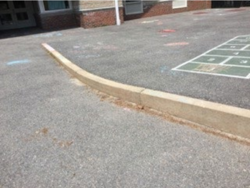
Fig. 1 Tripping Hazard on South Playground
