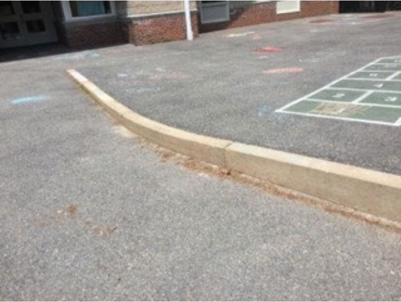
Fig. 1 Tripping Hazard on South Playground
