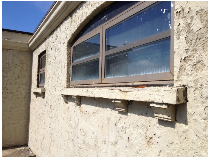
Typical historic window sills and replacement window
