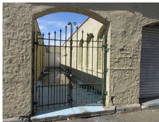
Central entry passage to bathhouse with blocked area drains
