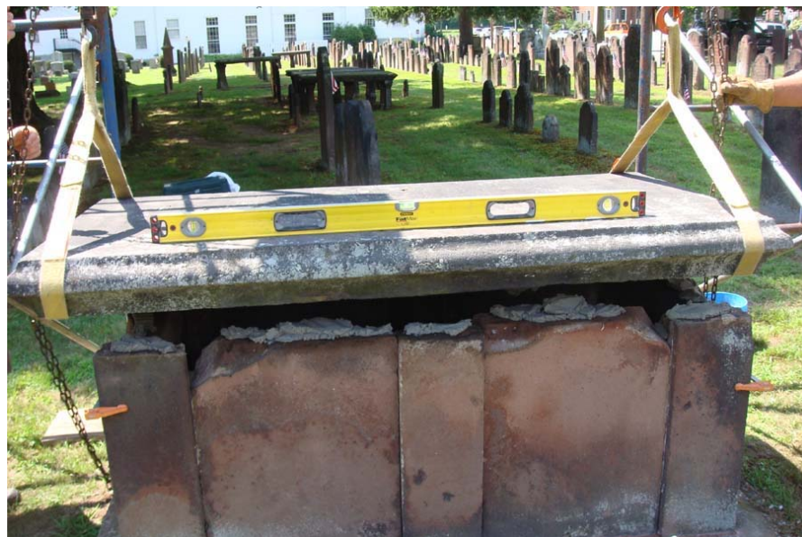
Example of re-setting a large ledger top with mortar onto tomb base with the aid of scaffolding and chain hoists
