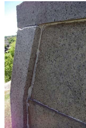
Old mortar and caulk
