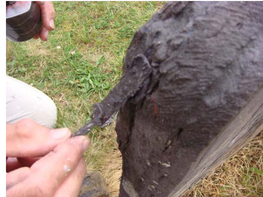
Filling top cavities with a pigmented crack filler by Sto. Excess material to be immediately wiped off with damp sponging
