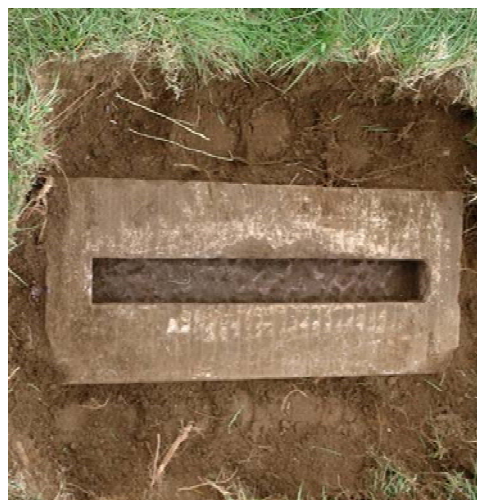
Old base reset higher and aligned with adjacent markers
