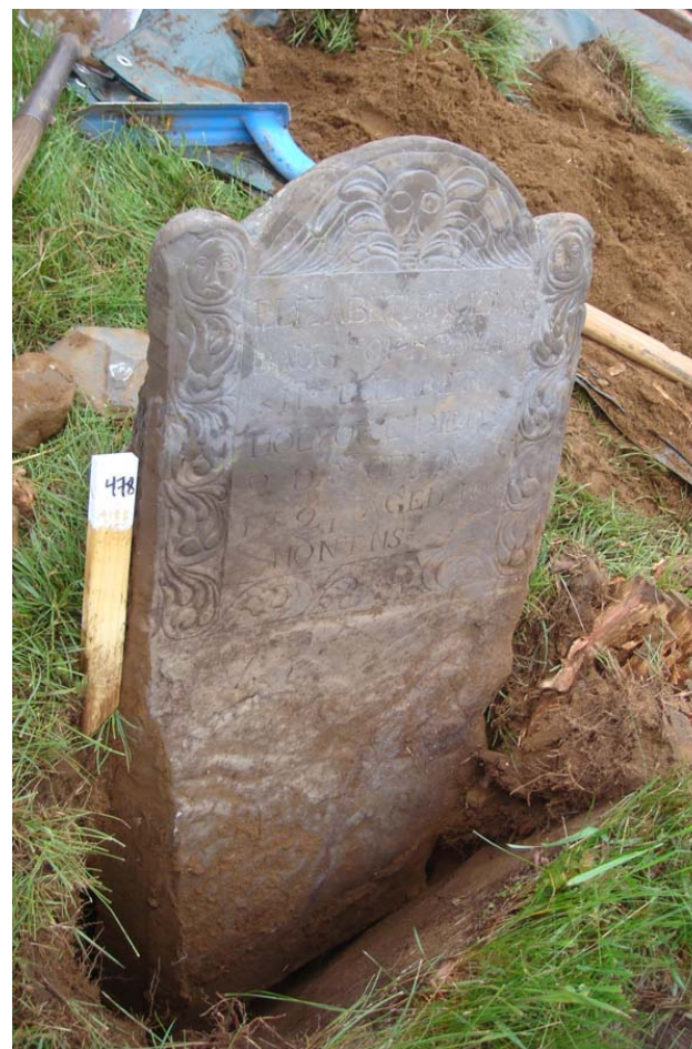
18th century markers often have as much below the ground as above. Only upon excavating this marker for resetting does the very massive below grade portion become apparent..
