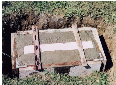
Poured base with form insert for setting slot
