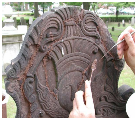
Filling cracks in a sandstone with a pigmented crack filler
