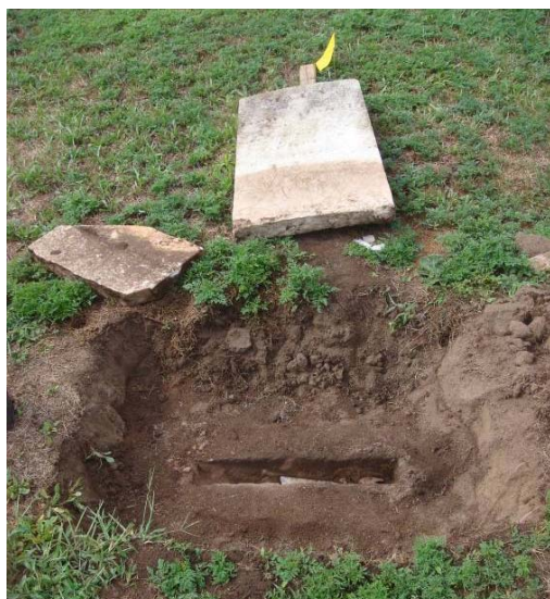
When excavating for resetting often original, or old bases are discovered
