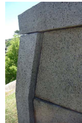
Joints cleaned with hand tools
