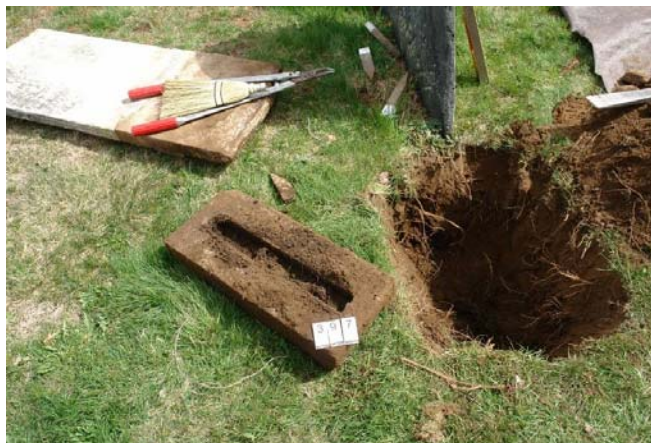
Old base removed and inspected for soundness
