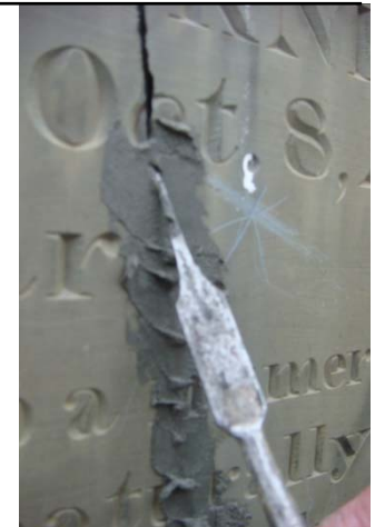
A pigmented Sto Crack Filler being tooled into an open face crack
