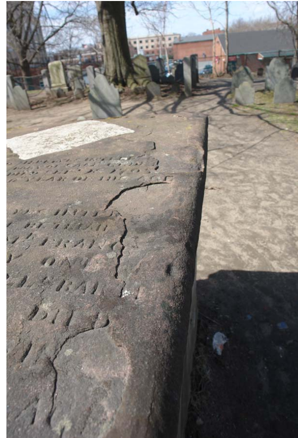
G4.1 Gedney Tomb. The top should be consolidated and after sufficient curing, losses and cracks filled with the appropriate materials.
