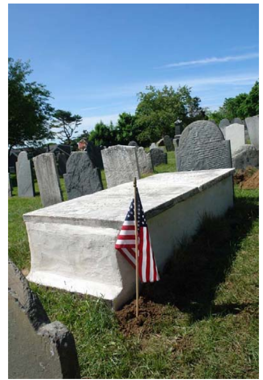
Before and after, New stucco applied to base (top restored)
