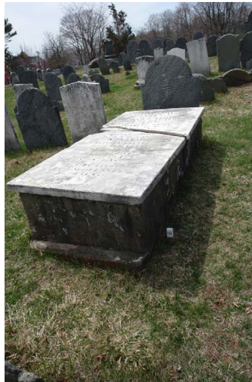
Before and after, New stucco applied to base (top restored)
