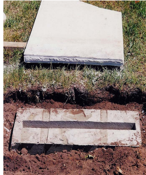
New base ready for resetting
