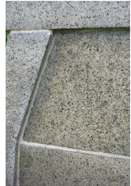
Example showing repointing with 1:1:6 with masonry sand
