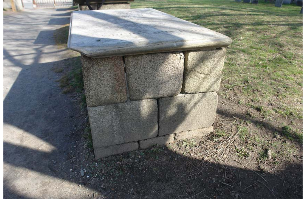
F2.2 Derby Tomb. This top will be reset with a pozzolanic hydraulic lime (typically #600 PHLc70 by Voidspan). The mortar can be removed if the tomb has to be dismantled in the future
