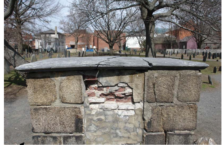
G7.1 Lynde Tomb. An example of priority “1”. Highly visible, deteriorating tomb with loose top fragments
