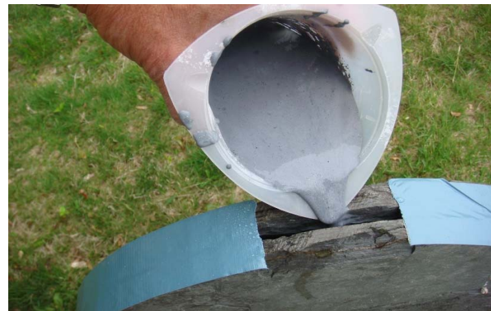
Filling voids with a pigmented flowable grout (VoidSpan PHLc)
