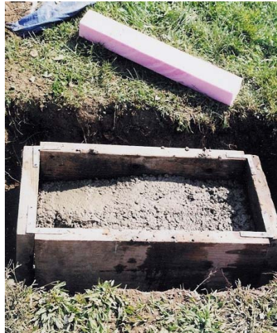
Formwork for new base
