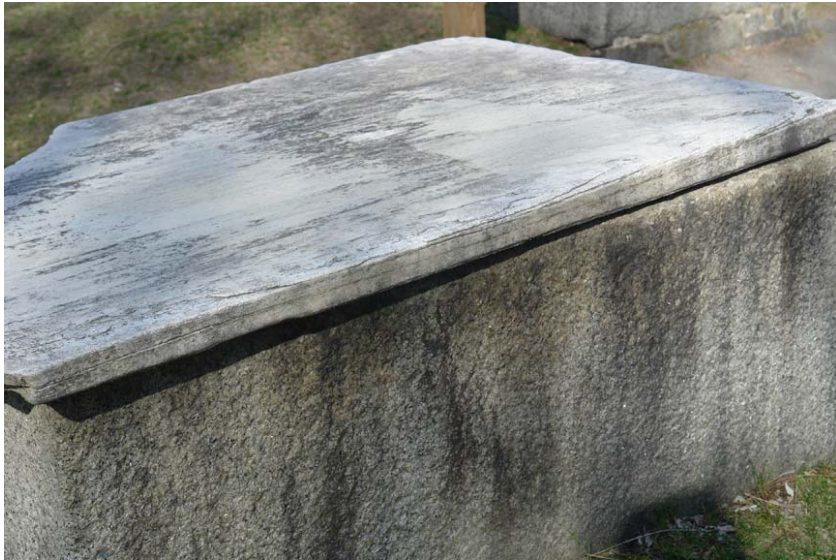
F1.1 Fisk Tomb This loose top can be secured to the solid granite base with a structural adhesive . There is little reason for it to ever be removed.
