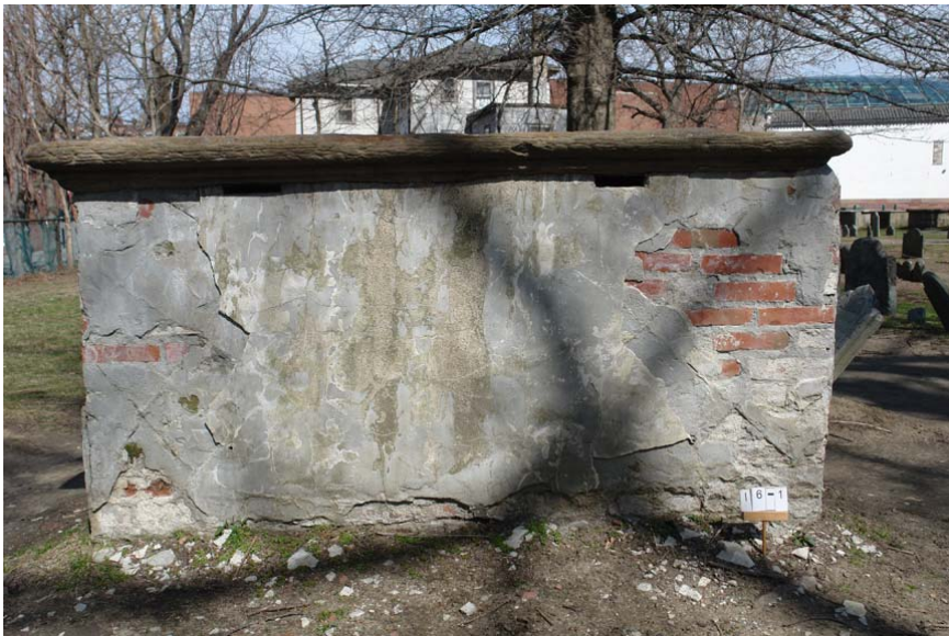
16.1 Bradstreet Tomb . Deteriorating stucco and loose top
