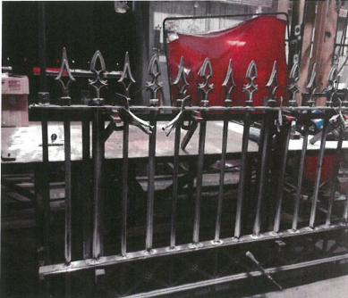
Original cast iron pieces are labeled, mapped, and then removed from the Common and taken to the foundry. At the foundry, the fence sections sandblasted to remove paint, repairs are made to the metal and then painted. The goal is to always keep as much of the original fabric of the fence as possible.
