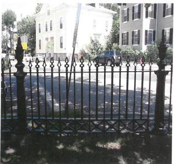
In both examples above, fence sections were completely missing and were recast in the original form. (Photos: CBI Consulting)
