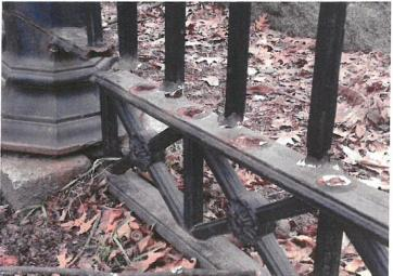
Above images (Photos: City of Salem): Missing fence sections along Washington Square East, bollards and fence section in need of repair and replacement at the Washington Street South entrance and severe structural damage to the existing fence example.
