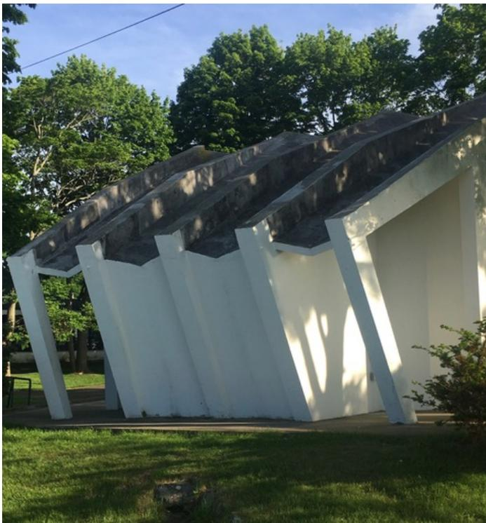
Looking southeast, the rear elevation of the shell, showing integrated concrete beams. 2018
