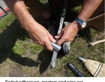
Failed adhesives, mortars and pins are carefully removed before proceeding with new conservation treatments. Mechanical removal was done with hand tools and, when required, smaller power tools.
