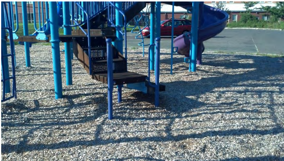
Settled Surfacing at transfer point
