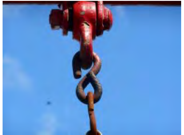
Swing hardware (s-hook, entanglement)
