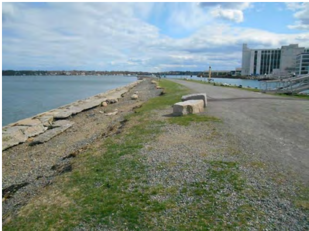
Erosion between path and see wall
