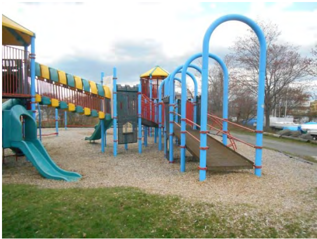
Accessible ramp into structure above surfacing
