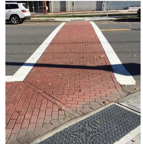
Imprint crosswalk – Colored asphalt
