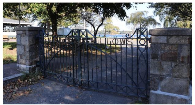
Gate, looking north, showing inconsistent treatment of mortars over time. 2018
