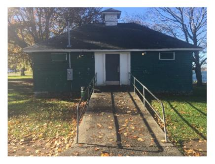
North elevation. In the 1950's, glass block sidelights (now boarded up) were added on either side of the main entrance. A recently added concrete ramp with metal railings provides accessibility. 2018
