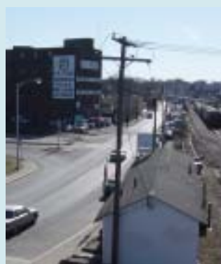
The reconstruction of Bridge Street offers the opportunity to create a well landscaped, quality road that will improve the identity of the corridor and enhance the edges of the park.
