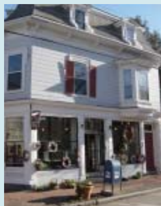
New development should be sensitive to the scale and character of the surrounding neighborhoods.
